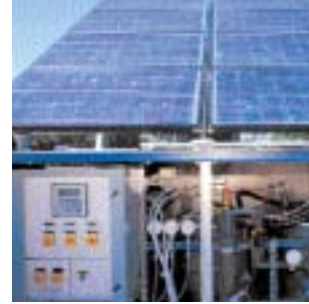
Photovoltaic cells rely on plastics' tough, weather resistant and light transmission properties to work effectively
